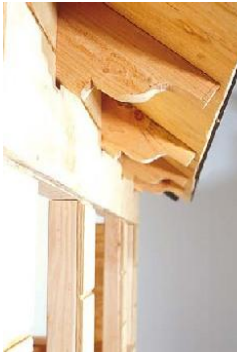
How to Build The Ace Clubhouse Steps Continued: 3 and 4
